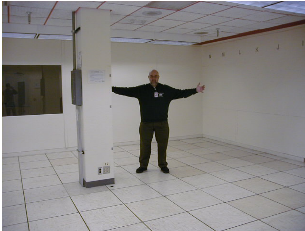
William F. Slater, III Data Center Manager, BP Naperville Data Center, December 2005
