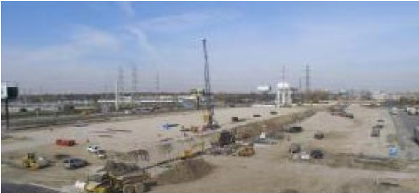
The site of Microsoft's data center project in Northlake, Ill.
