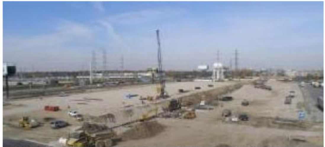
The site of Microsoft's data center project in Northlake, Ill.
