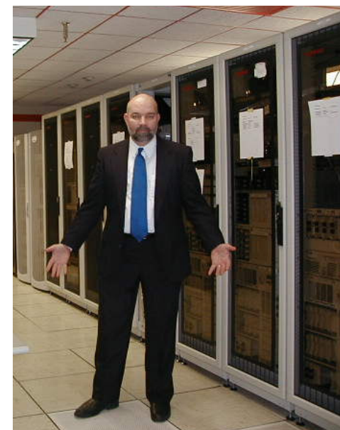
William F. Slater, III Data Center Manager, BP Naperville Data Center, October 2002
